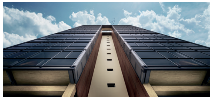
"TREET" IN BERGEN, NORWAY, THE WORLD'S TALLEST WOODEN HOUSE – 52 METERS HIGH AND 14 STOREYS. TEKNOS HAS SUPPLIED TEKNOS FR FAÇADE AND TEKNOS FR PANEL.
