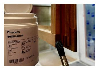
Teknoseal 4000 applied by brush to exposed end grain as part of the finishing process
