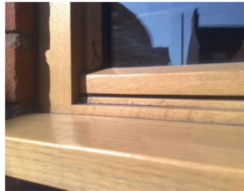
Gaps and exposed end grain should be sealed with TEKNOSEAL products before the coating is reapplied.
