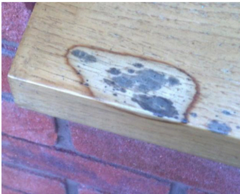
Localised staining can be sanded out using a detail sander and the coating system reinstated.
