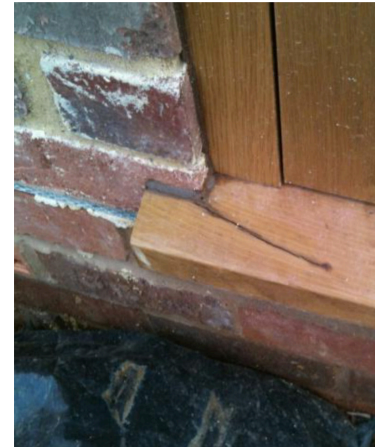
The surface of oak joinery tends to split in service, disrupting the protective coating, allowing water to enter and react with Tannic Acid
