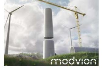
Modvion's innovative wooden turbine towers' glulam modules are coated with polyurea for various advantages: it improves mechanical protection, and most importantly for this object, it brings waterproofing and weather resistance.
