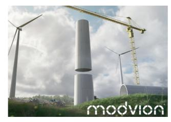
Modvion's innovative wooden turbine towers' glulam modules are coated with polyurea for various advantages: it improves mechanical protection, and most importantly for this object, it brings waterproofing and weather resistance.
