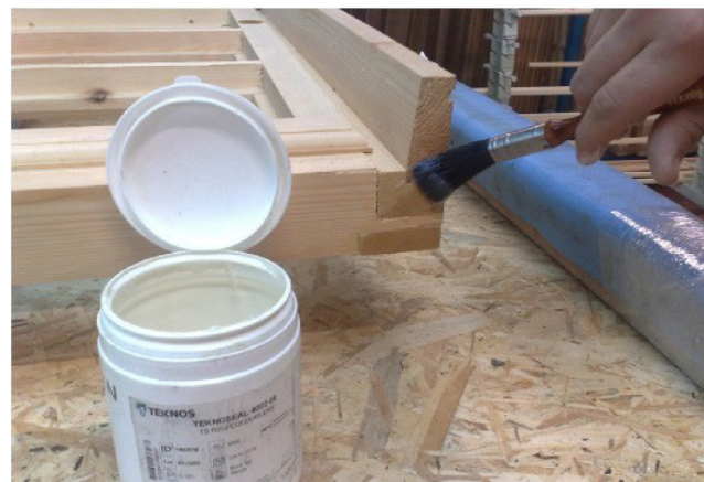
TEKNOSEAL 4000 applied by brush to exposed end grain, after preservative treatment
