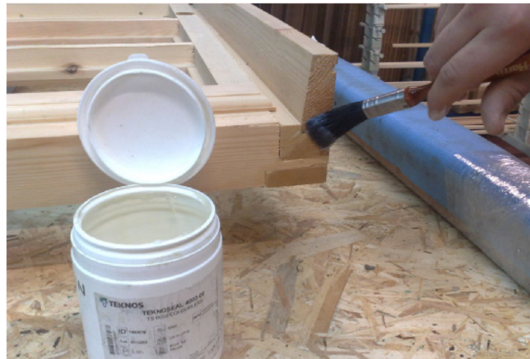
Teknoseal 4000 applied by brush to exposed end grain prior to factory finishing
