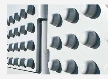
nstead of welding rolled shells for large, bulky, cylindrical tower elements that are to be transported at full length on large, heavy-duty semi-trailer flatbed trucks, Andresen Towers started producing many different long, bent steel segments that can be transported to the end destination cheaper and faster on normal platform trucks. The steel segments allow hub heights of more than 100 meters, because they are bolted together into towers directly on site.
