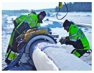
**INFRALIT EP 8064** Powder Coating is Fusion Bonded Epoxy (FBE) for field joint system with Wehocoat device. TDS No. 1593.
