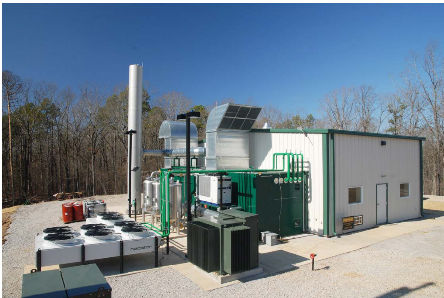
Soundproof special containers for cogeneration units are painted by Wenker.
