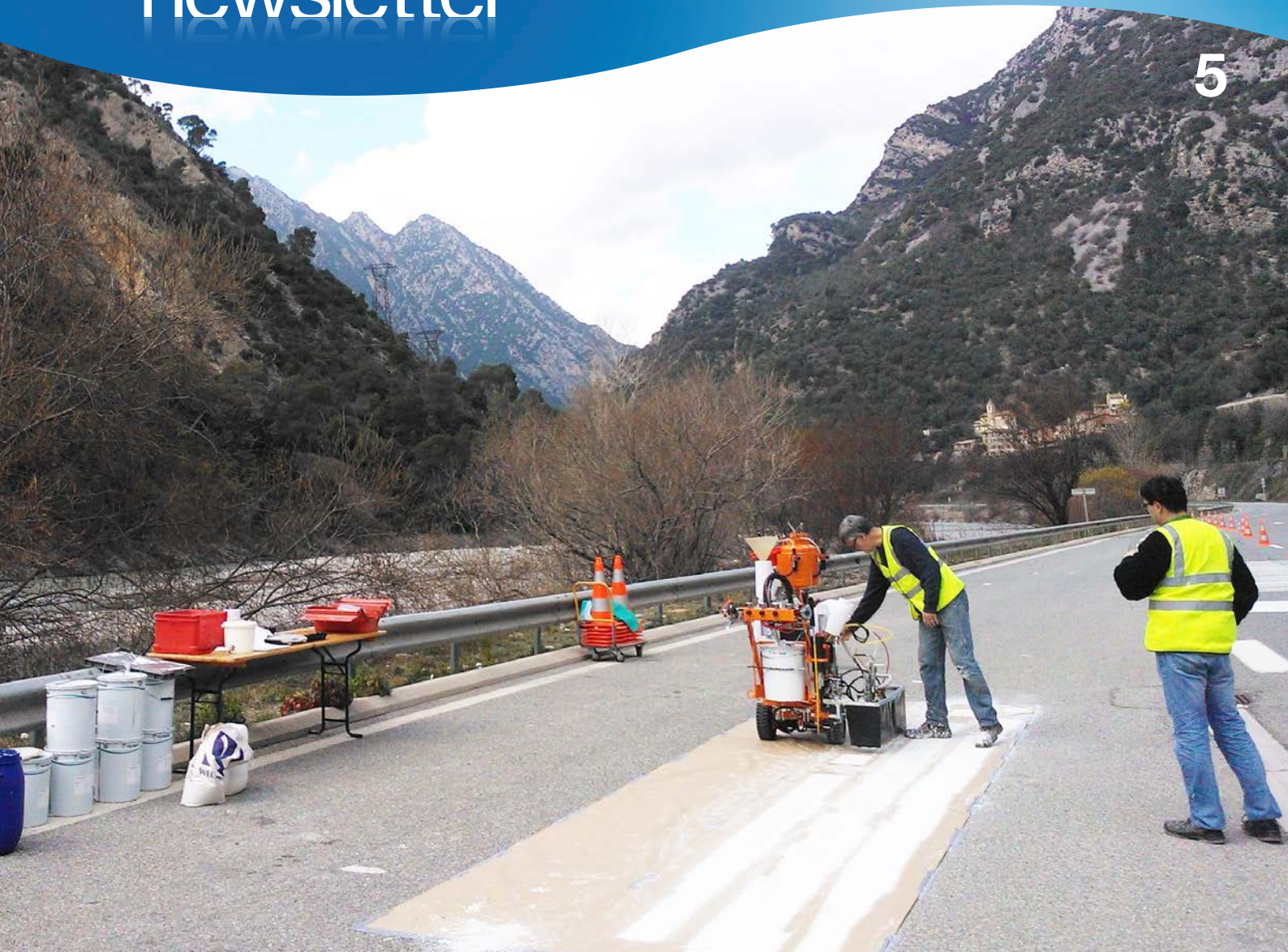
Test painting with the new water-borne TEKNOROAD 3058 road-marking paint was performed on surfaces such as mountain roads last winter.
