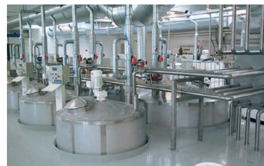
With R&D, production and technical staff all under one roof, response time is fast.
